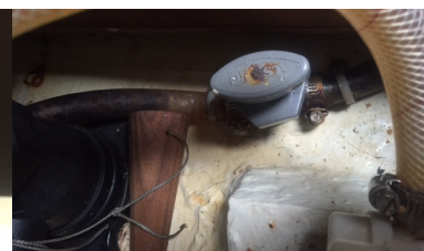
Ice Box Drain under galley sink
